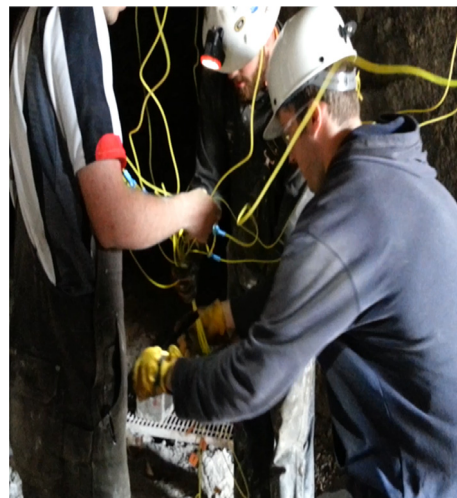
(d) Connecting individual detonating cords together.
